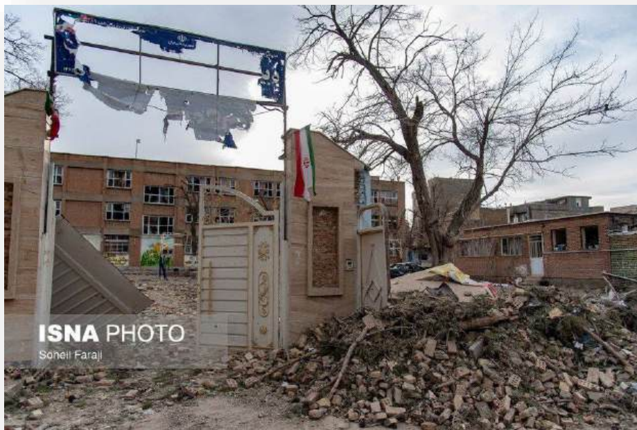
The Imam Reza boys' school in Abyek, Qazvin, was seriously damaged. An innocent schoolboy was killed and 3 of his schoolmates were injured.
